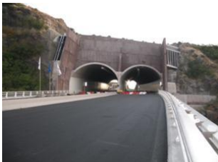
The covered trench after works
